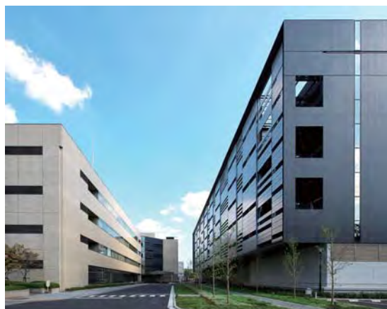
MCC Mitaka Building: North Block (left) and South Block(right)
